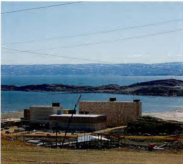
Construction site of the Baffin Regional Hospital, Iqaluit, Nunavut.
