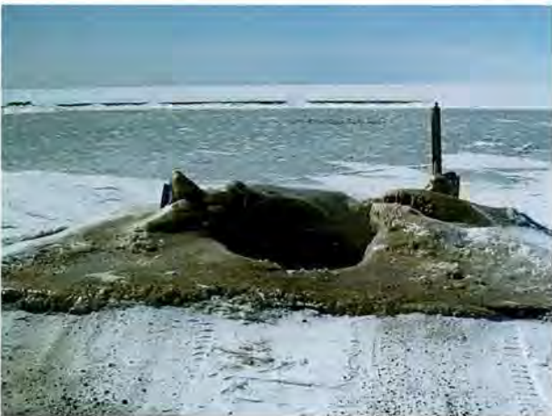
Sewage disposal site, Arviat, Nunavut
